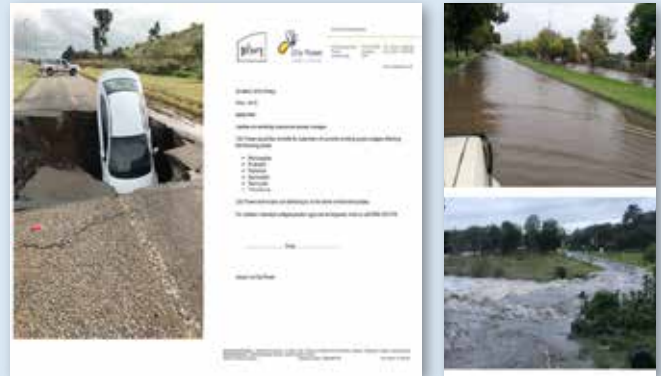
Figure 6: Left: Flooding of railway underpass on Nellmapius Drive, Irene, Pretoria where the road was subsequently officially closed on 23 March 2018 (source: ENCA). Right: A large sinkhole due to heavy rains on the R55 leading to Valhalla, Centurion, Pretoria on 23 March 2018 (source: Tshwane Metro Police – Twitter)
